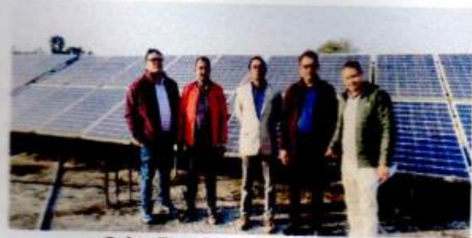
Solar Panels on the roof-top
