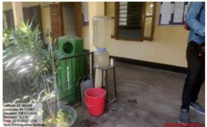
Drinking Water Facility
