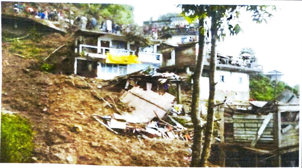
Figure 12: House Collapsed Due to Landslide from heavy rainfall
