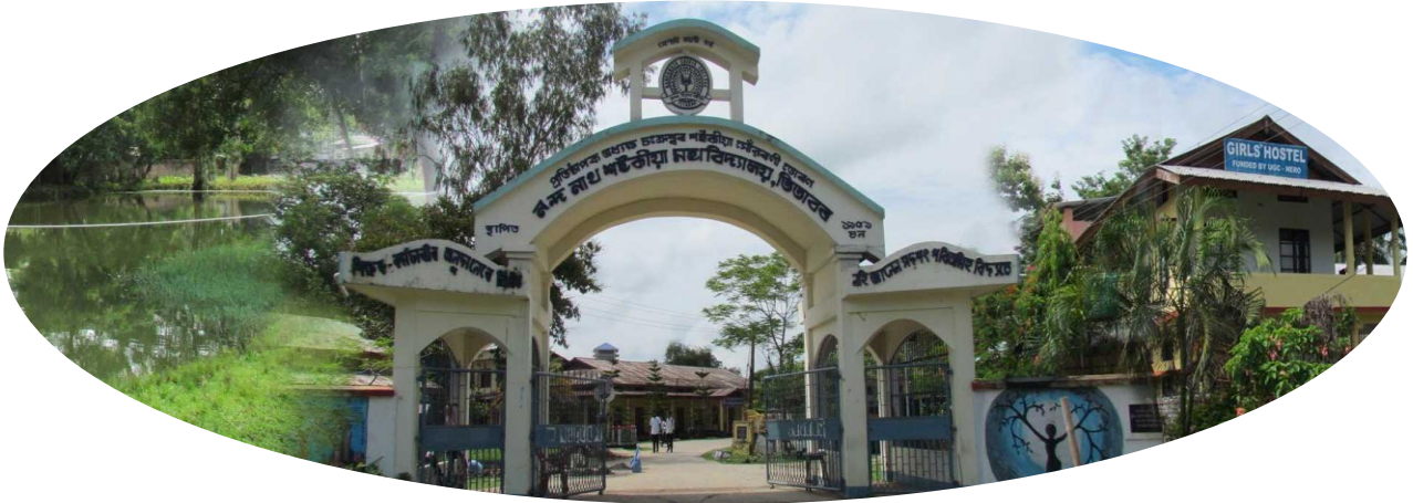
Main Gate of the College (Front View)
